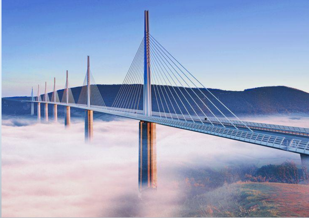
Millau Viaduct, France
